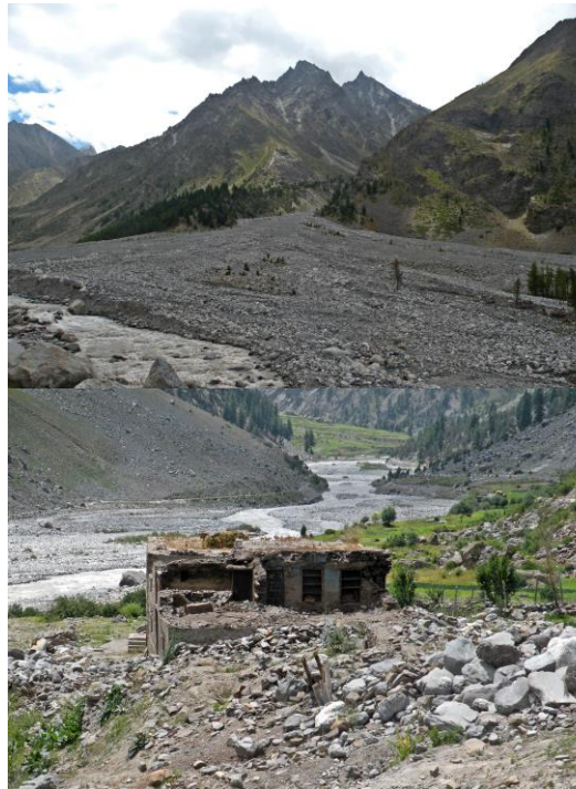
The 2013 cloud burst caused widespread damage to property and livestock in Miyar valley
